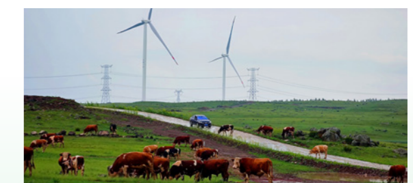
→ CGN's Xinsheng Wind Farm delivering green electricity for Beijing 2022
