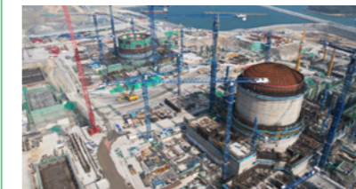
Construction site of Taipingling NPP, Guangdong
