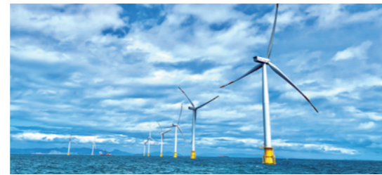
→ Dalian offshore wind farm in Pingtan
