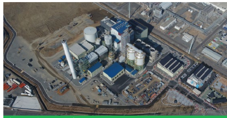
The Daesan Biomass Power Plant
