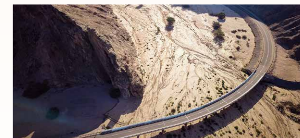
21 km mine road invested and constructed in Namibia
